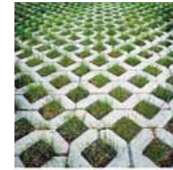
Recharge zones with grass paver blocks to increase percolation of water into the soil for water recharge and reuse of the wells
